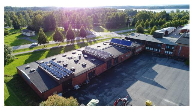
Multiple solar collectors and solar thermal panels were deployed on the Ikaalinen office building in autumn 2017. The exceptionally cold beginning of the year, as well as the warm and sunny summer, has been an excellent time for versatile testing and control of the solar and smart thermostat system.
